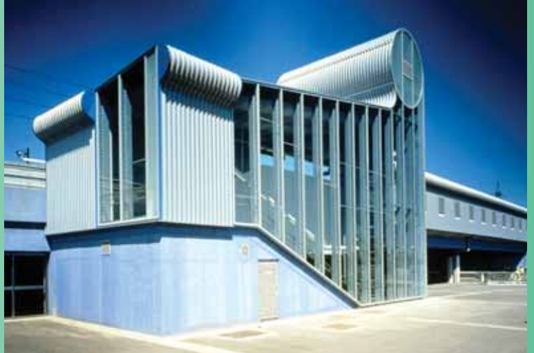
Entire surface perforated
