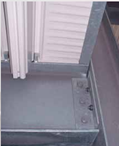
Positioning of trapezoidal profiles by using steel cleats.
