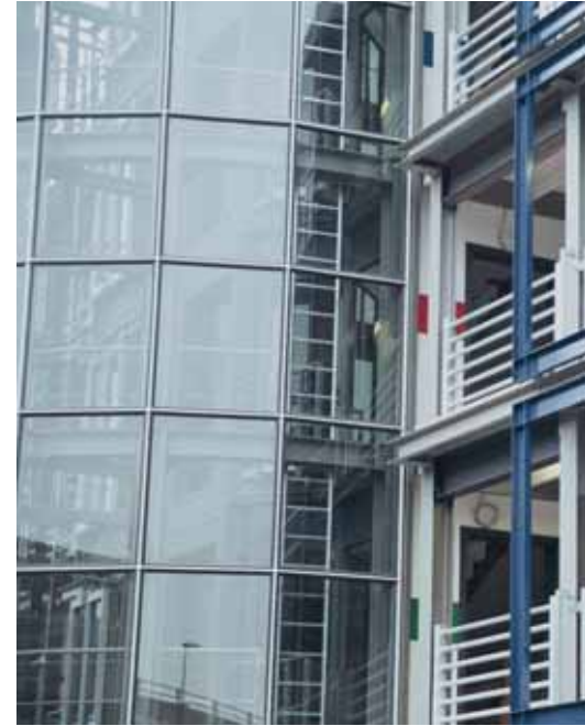
Car park in service
