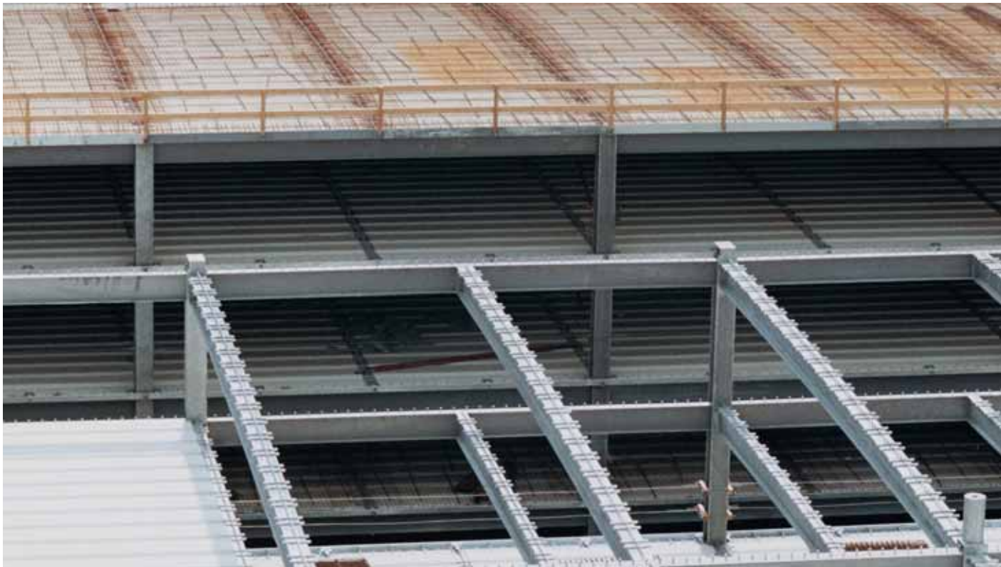
Parking deck in steel composite construction, mounting phase.
