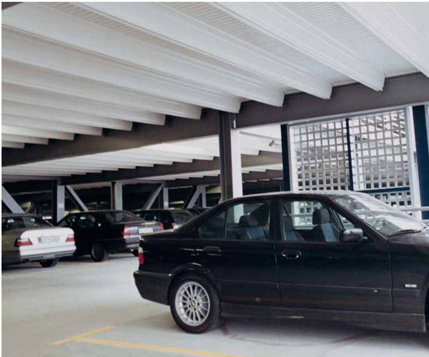
Parking deck in steel composite construction.
