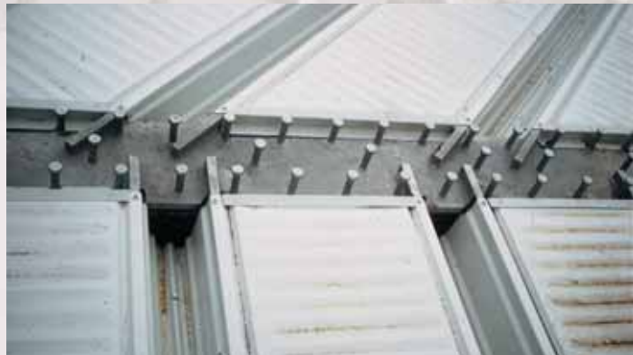
Easy diagonal positioning of Hoesch Additive Floor®.
